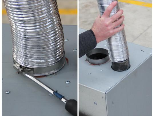
**WARNING:** The flue connection **MUST** be secured with the clips provided and tape **MUST NOT BE USED**. If any of the flue pipe is damaged and integrity compromised then it should not be repaired with tape, it should be replaced.
