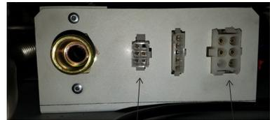
**If you do not connect the powerflue electrical cable to both the fireplace and the powerflue, this will result in an error when the fireplace is turned on.
