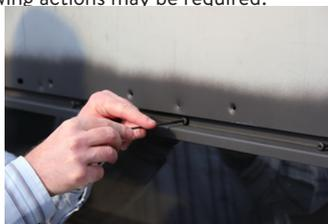
**Step 1:** Remove fascia panel (if fitted) by pulling it from the wall.
